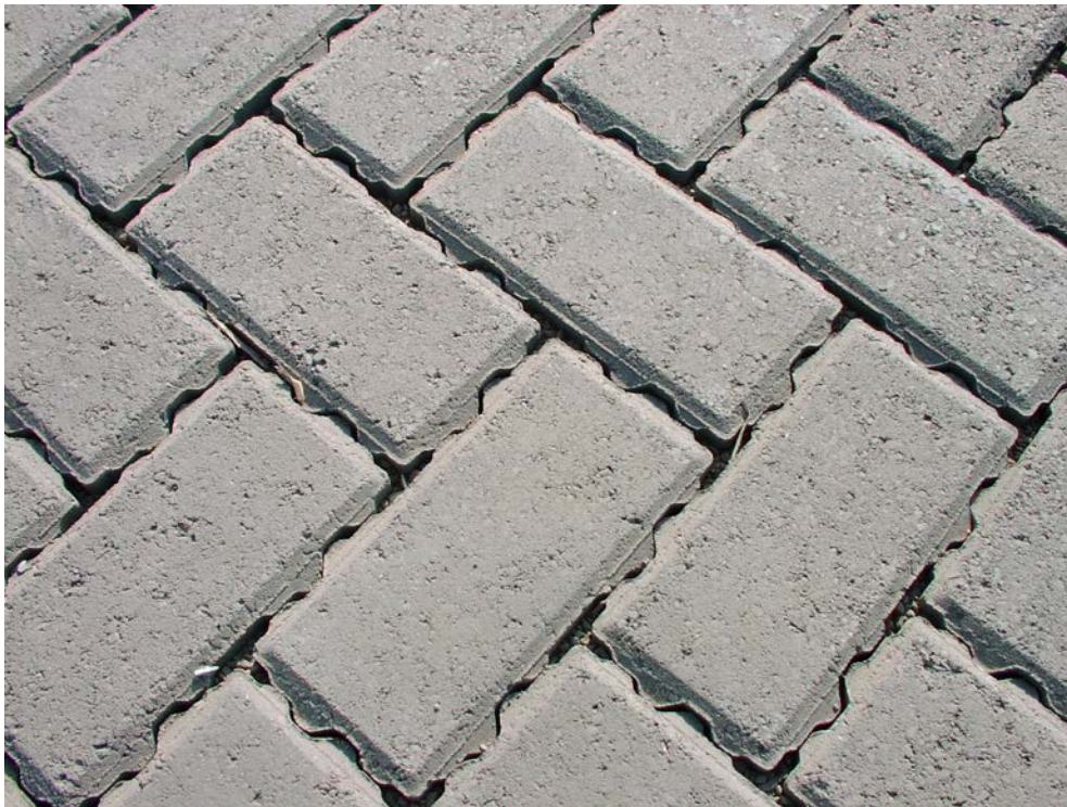
Figure 1. Priora Permeable pavers installed in herringbone pattern
