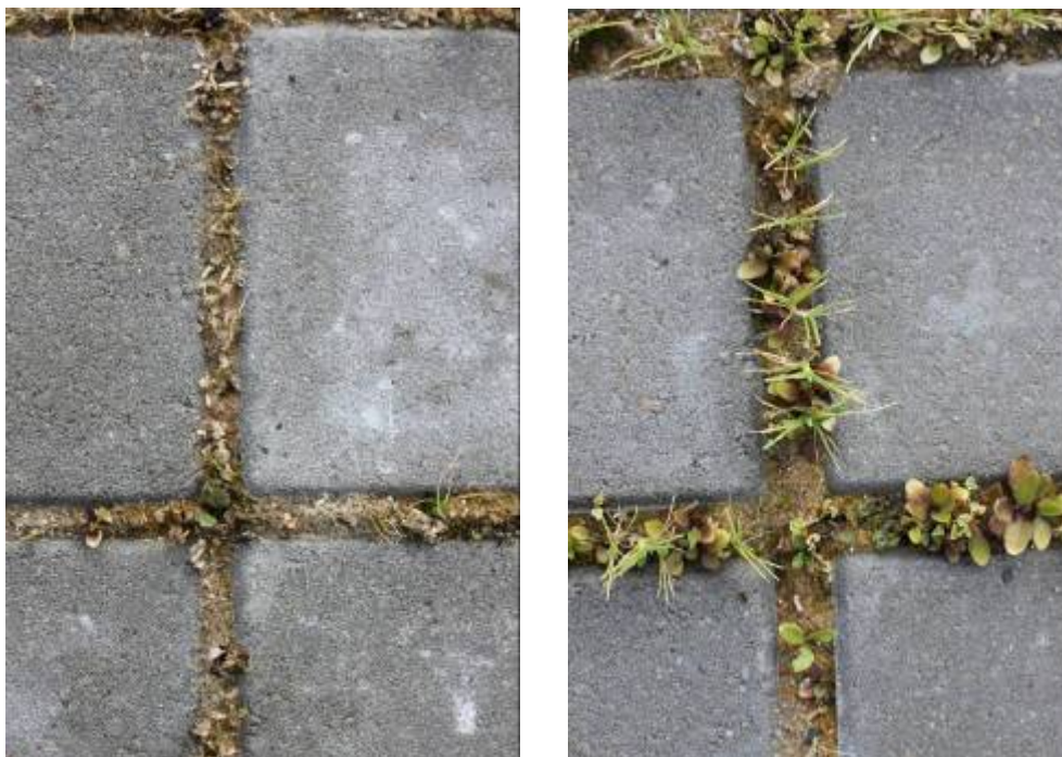
Figure 7 – Impact of joint width on weed coverage in “mini” paving trial, for pure sea sand. Left: 3mm; Right: 11mm
