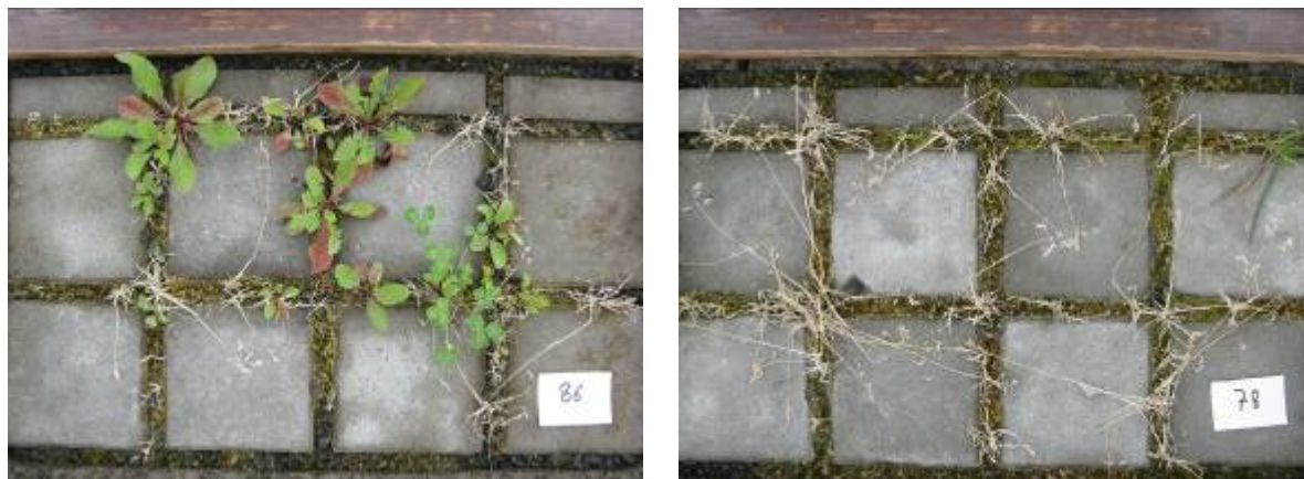
Figure 8 – Impact of type of paving bed on weed growth in “mini” paving trial. Polluted joint filler of limestone 0/6.3 in wide joints (11 mm). Left: closed paving bed (limestone 0/6.3); Right: open paving bed (porphyry 2/6.3).
