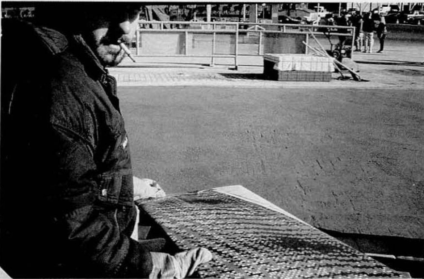
Figure 14. The pattern was transferred to the plans so they could be followed by the contractor. Figura 14. El patrón fué transferido a los planos para que pudiera ser seguido por el contratista.
