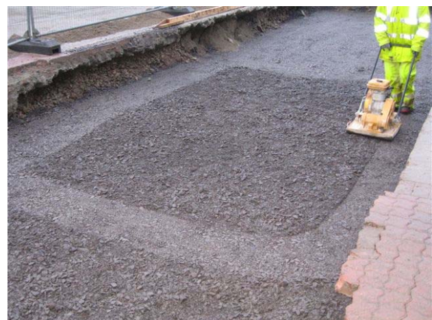
Figure 5. 150mm thickness of compacted Capping Material was installed throughout the test zone prior to installing polythene tanking.
