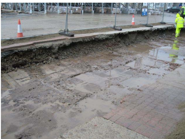
Figure 4. The test area has been excavated to reveal alluvium clay with a California Bearing Ratio of 5%.
