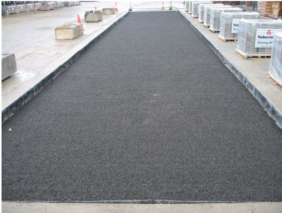
Figure 8. Prior to the laying of pavers, a 50mm thick course of 6mm single sized grit was installed in each Test Item.
