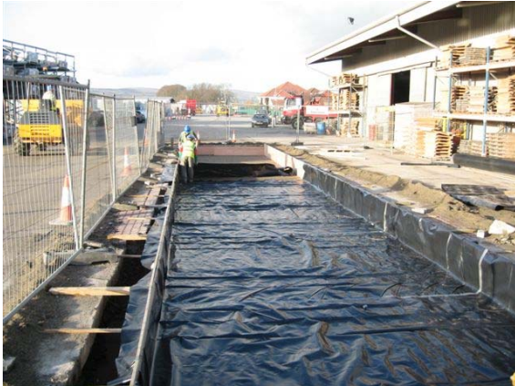
Figure 6 (left). 2000 gauge polythene was installed to achieve tanked conditions for each Test Item. Figure 7 (right). Test Item 4 required the installation of two layers of a geogrid material known as Tensar SS40. The lower layer is shown here directly over the polythene membrane. The second layer was installed between two courses of Coarse Graded Aggregate..
