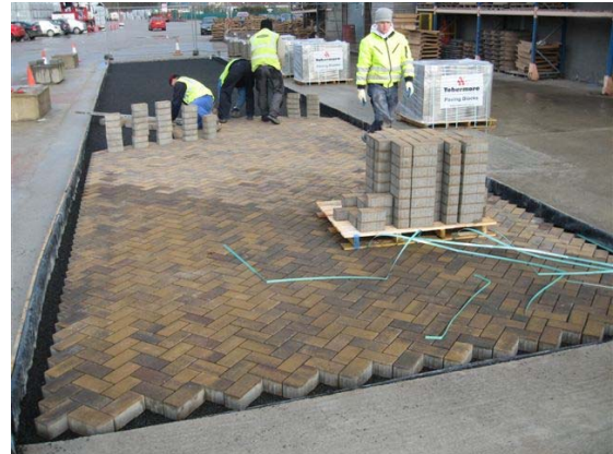
Figure 9. Permeable pavers were installed to a 45° herringbone pattern.
