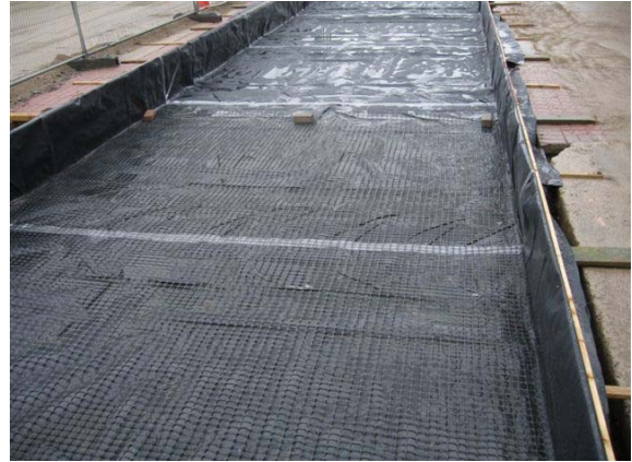
Figure 6 (left). 2000 gauge polythene was installed to achieve tanked conditions for each Test Item. Figure 7 (right). Test Item 4 required the installation of two layers of a geogrid material known as Tensar SS40. The lower layer is shown here directly over the polythene membrane. The second layer was installed between two courses of Coarse Graded Aggregate..
