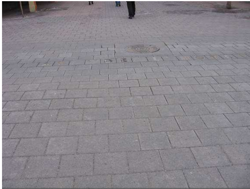
Figure 1. Prince-Arthur Street at the corner of Hôtel-de-Ville Street in Montreal, QC. This section, exposed to traffic, was built in 1996 with 300 x 300 x 100 mm thick pavers (Source: City of Montreal)
