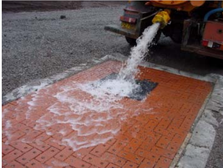
Figure 5. Trial pavement filled with water prior to testing.
