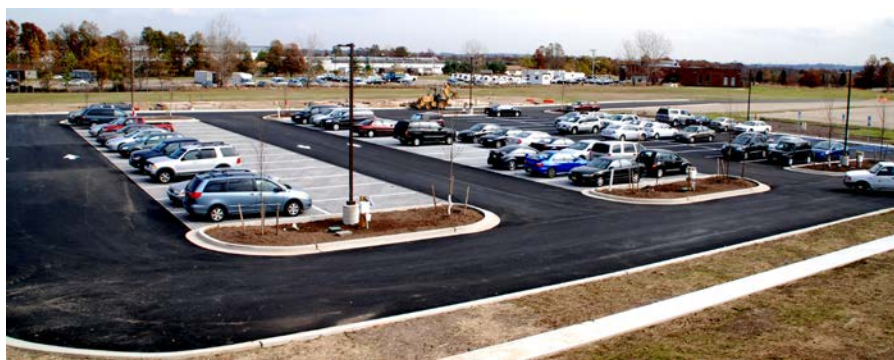
Figure 4. Pervious concrete (light colored parking area on left), PICP (center) and porous asphalt (right) at a test facility at US EPA laboratories in Edison, New Jersey
