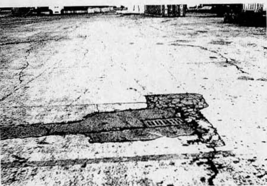
Figure 12: Cracking of in-situ concrete construction.
