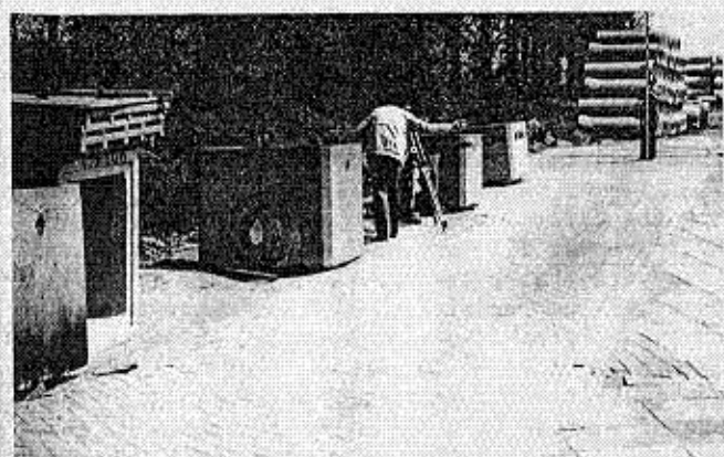
Figure 13. Level measurement (pavement I, 10-5-'83).
