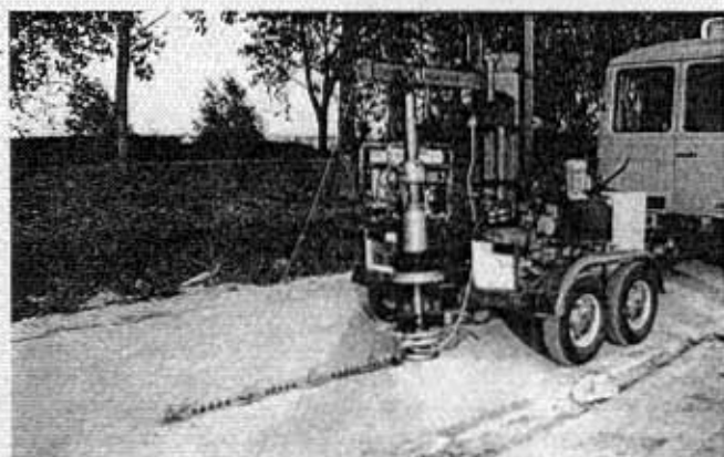
Figure 10. Falling-weight deflection measurement (pavement I, 4-10-'82).
