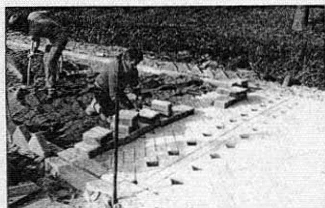
Figure 6. Road paving in accordance with the traditional craft method.
