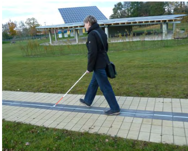
Bild 2. Leitstreifen in einem Gehweg im Klimapark Rietberg / Illuminated linear guidance system integrated into a footpath at Klimapark Rietberg
