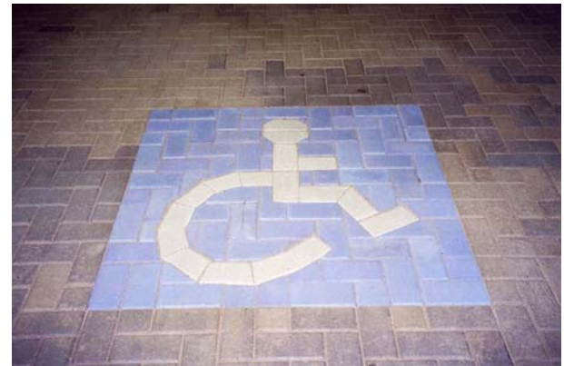
Figures 7 and 8. Disabled parking bays formed with reflective units.
