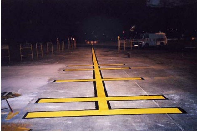
Figure 9. Apron 'Stop bars' formed using reflective material.
