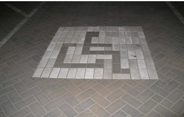
Figures 7 and 8. Disabled parking bays formed with reflective units.
