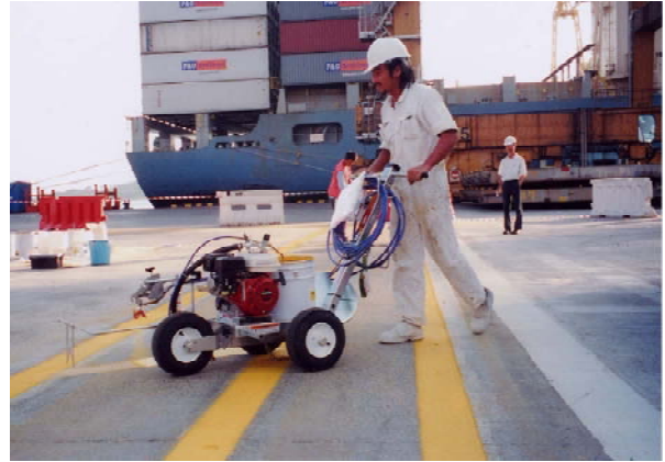
Figure 10. Reflective mix application.
