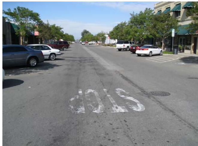
Figure 2: Faded markings on asphalt road
