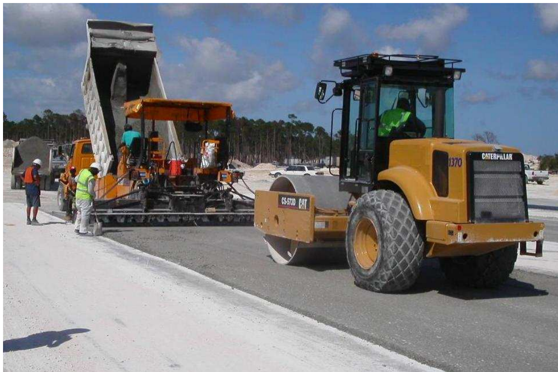
Figure 2. Infilling and compacting using 'hit and miss' method.
