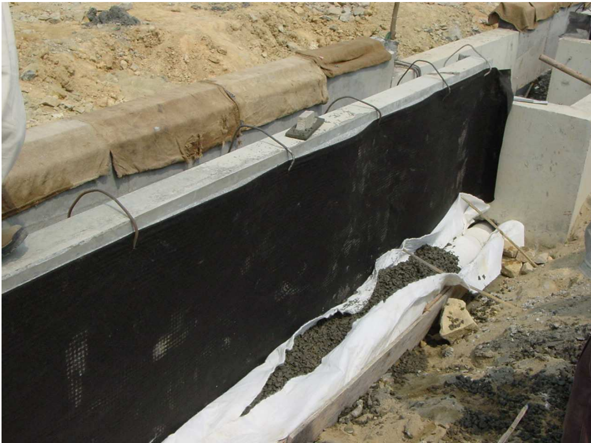
Figure 7. Bedding layer drainage detail.
