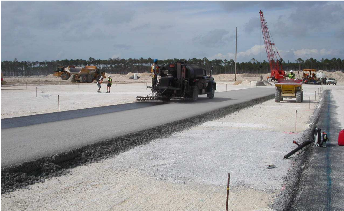
Figure 5. Application of Bitumen Curing Layer.
