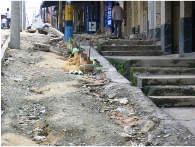
Figure 14. Early stages of construction.
