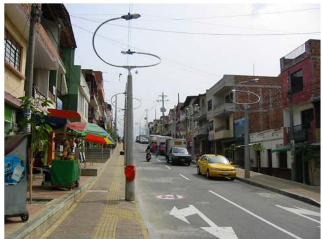
Figure 5. After: Well-defined circulation with concrete pavers.
