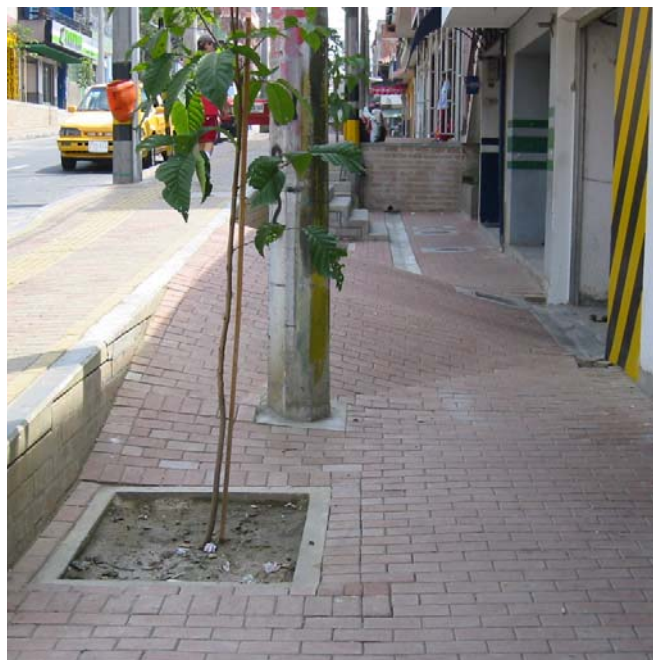
Figure 29. A few accesses had to be solved.
