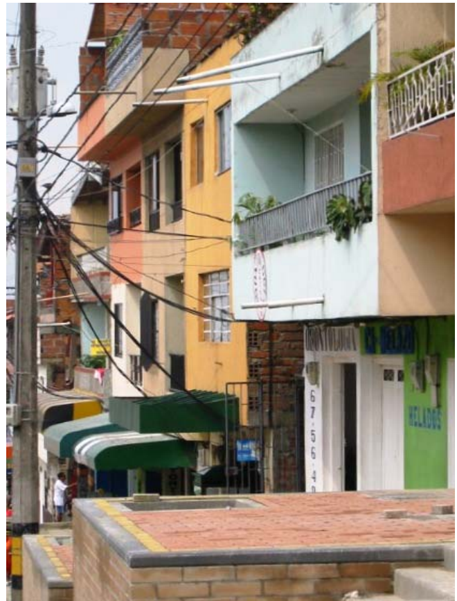
Figure 23. Roof drains onto a terrace.
