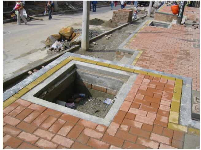
Figure 19. The small unit module in action.
