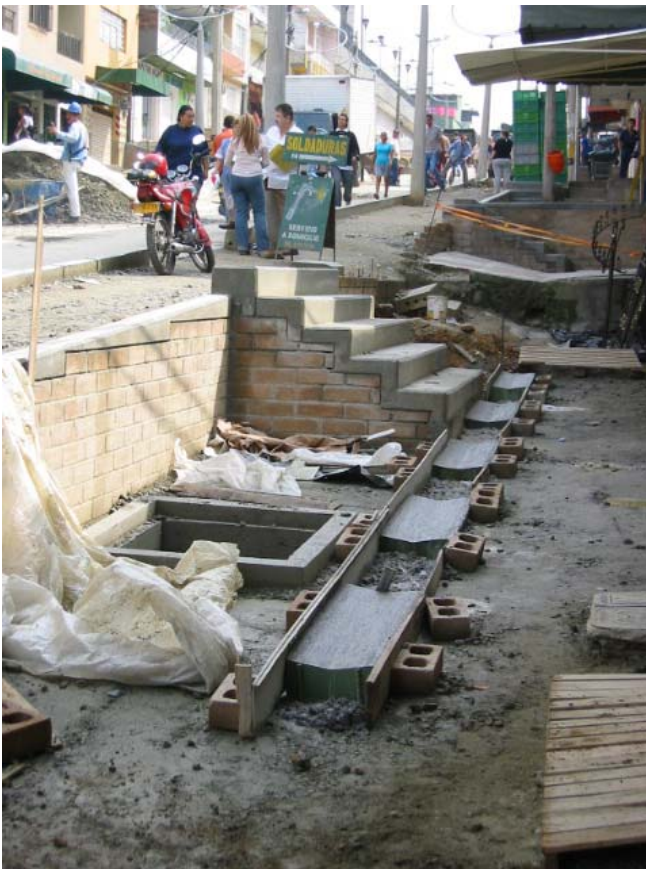
Figure 16. Drainage in progress.
