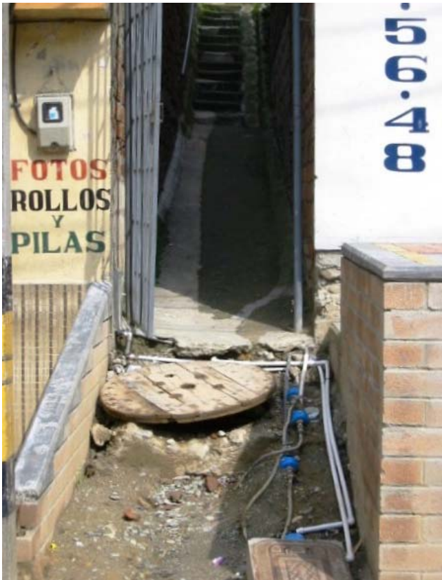
Figure 10. Typical entrance under renovation.
