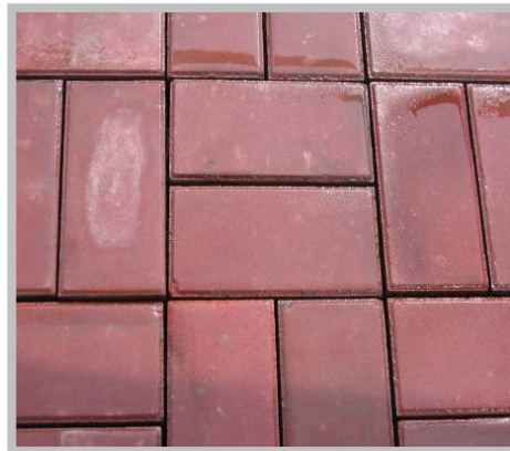
Fig. 7 - IPS used as permeable paving
