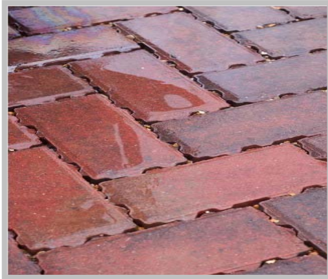
Fig. 6 - Typical permeable paving
