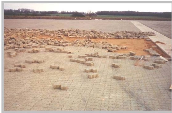
Fig. 2 – Displacement of blocks
