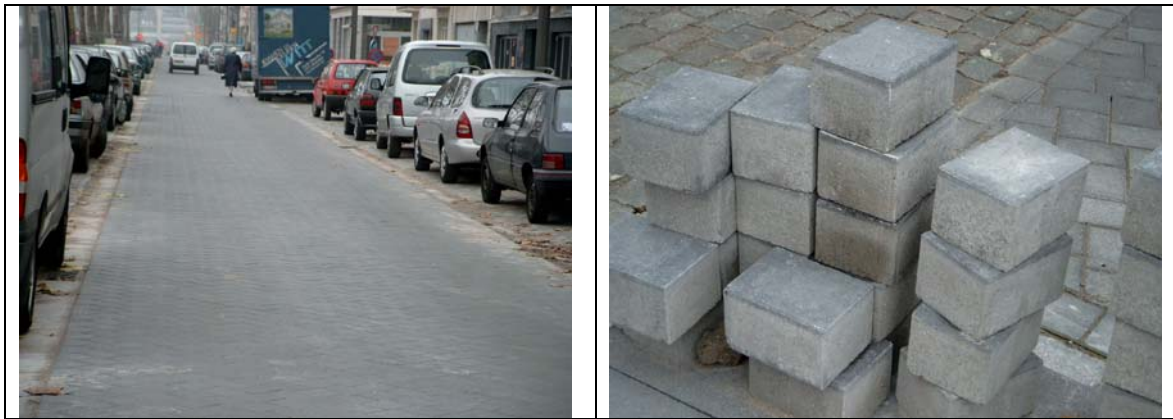
Figure 5. Separate parking lanes at the Leien of Antwerp with photocatalytic pavement blocks
