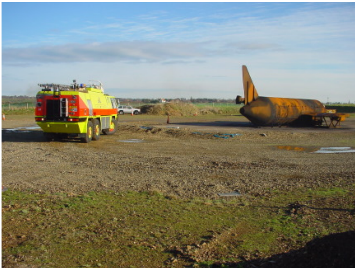
Figure 1. The original Fire Training Ground at Jersey Airport. Water, foam and other contaminants can permeate into the ground and pollute watercourses and the aquifer below.
