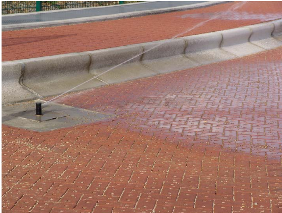
Figure 6. When environmental and operational conditions are suitable, water is sprayed over the pavers from where it evaporates.
