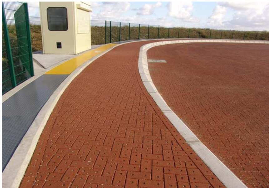
Figure 5. The fire chief controls training events from the control centre located on the perimeter of the new fire training ground.
