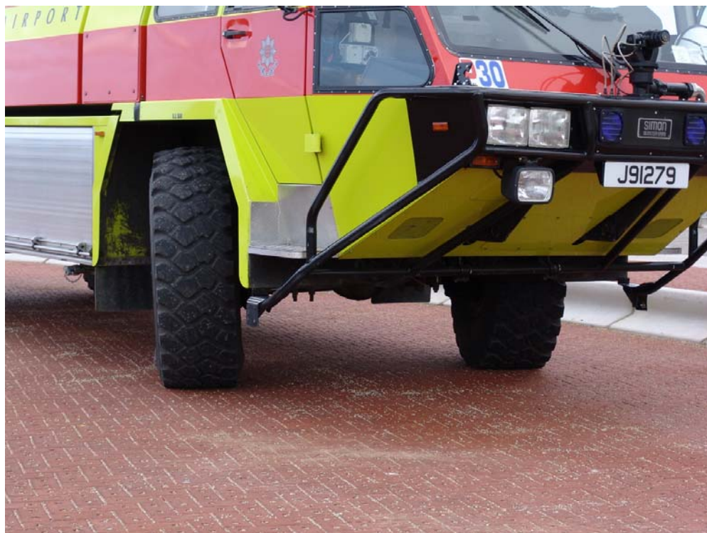
Figure 11. The pre-construction trials confirmed the suitability of the paving system for 12t axle fire trucks.
