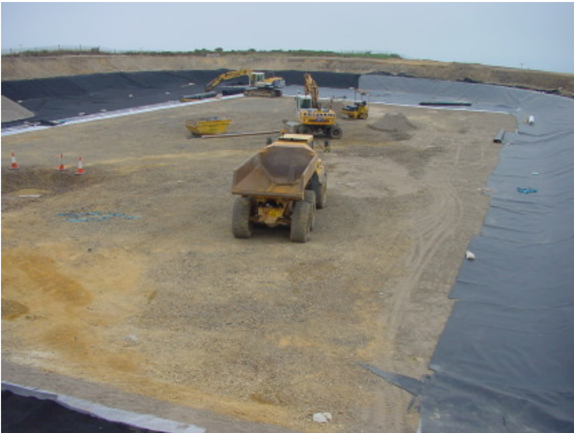
Figure 2. The contaminated material has been excavated and the lining to the evaporative cell is being installed.
