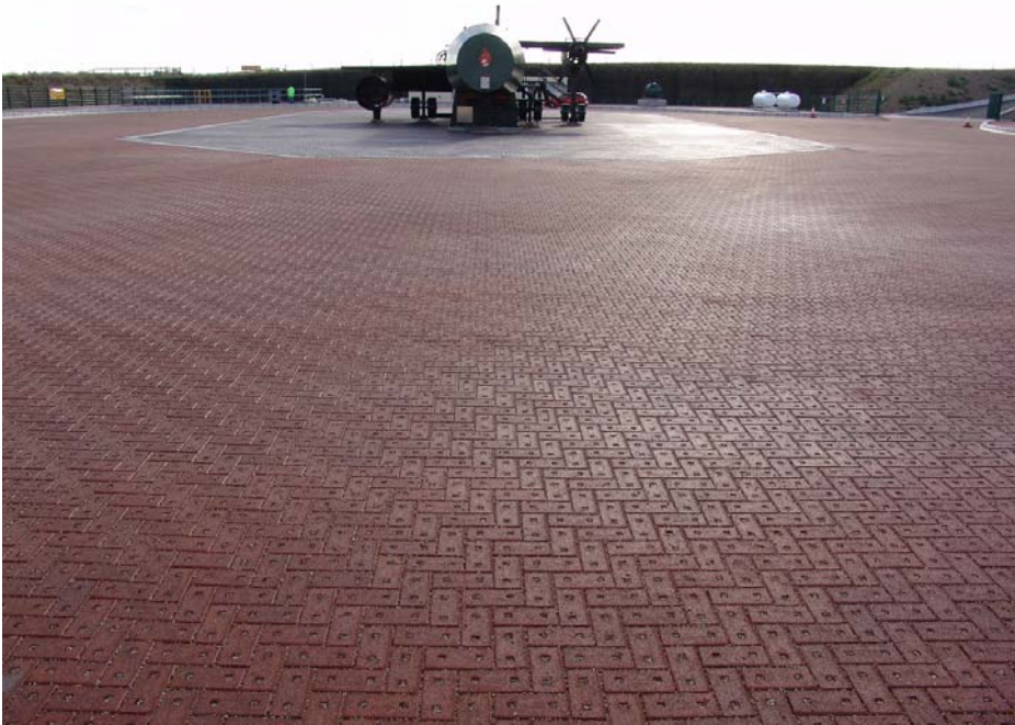
Figure 4. The inner zone pavers drain to a holding tank where dirty water is managed. The outer pavers are permeable allowing all the winter's rain to be stored in readiness for summer evaporation.
