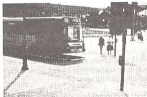
Figure 6. Victoria Road, Hartlepool, UK, showing high quality pavers on steel fibre reinforced concrete base.
