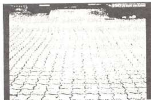
Figure 7. Failure of surfacing on a car park deck as a result of jointing sand being washed/vibrated into bedding course.
