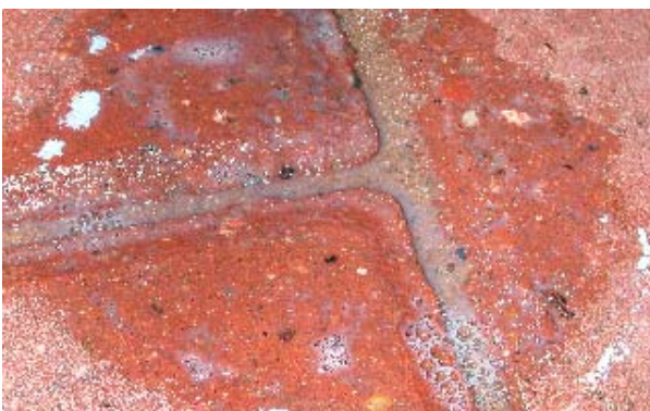
Photograph 6. Water and uncured stabiliser.
