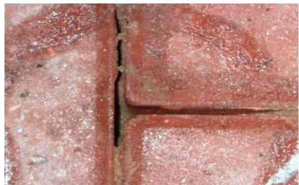
Photograph 7. Joints sucked out.
