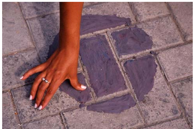
Photo 2. Sealing the paver's surface.
