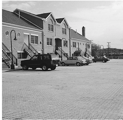
Figure 2. Concrete pavers support vehicular traffic and parking over a concrete parking structure next to a residential development.
