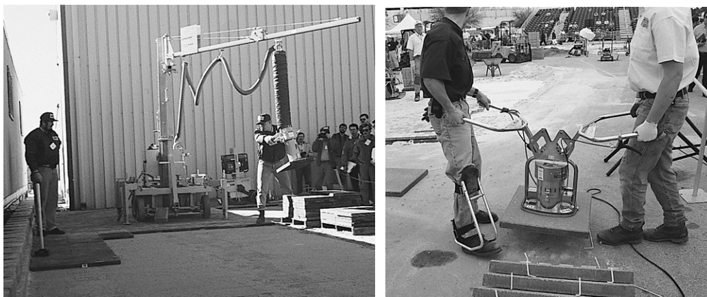
Figure 17. Vacuum assisted mechanical equipment for installing paving slabs.
