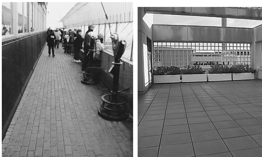
Figure 1. Concrete pavers provide a durable and attractive roof surface. At left is the observation deck of the 86 th floor of the Empire State Building in New York City. At right is a hotel plaza deck constructed with concrete paving slabs.
