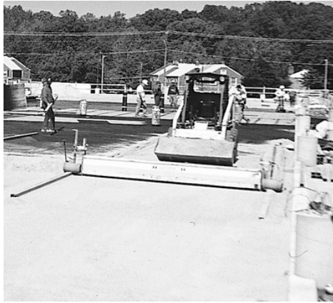
Figure 15. A mechanical screed used to level bedding sand on a roof parking deck project.
