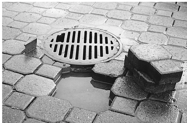
Figure 12. An absence of holes in the sides of this roof drain led to ponding.
