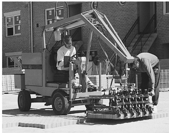
Figure 16. Mechanical equipment used to install concrete pavers on a roof deck.
